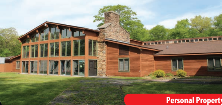
25,068 Sq. Ft. Main Office/Administration Building
