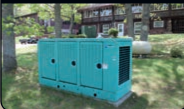
85KW CUMMINS GENERATOR
