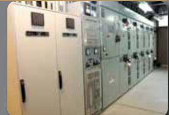
13.8 KV TRANSFORMER / 4160 V TRANSFORMER / 13.8 KV, 4160 V, 480 TRANSFER SWITCHES / 4160 V MOTOR CONTROL CENTERS
