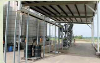
262,000± GALLONS OF TANK CAPACITY, SOME INSULATED W/HEAT, SOME AGITATED, CONCRETE CONTAINMENT WALLS
