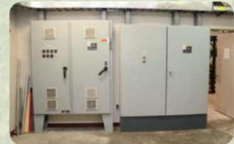
1,000 KVA TRANSFORMER FEEDING 480V ALLEN BRADLEY CENTERLINE 2100 MOTOR CONTROL CENTER, SQUARE D QED 1,000 AMP SWITCHBOARD
