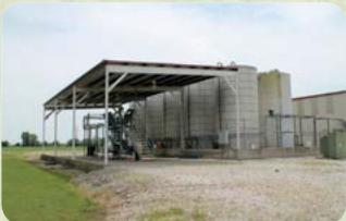
262,000± GALLONS OF TANK CAPACITY, SOME INSULATED W/HEAT, SOME AGITATED, CONCRETE CONTAINMENT WALLS
